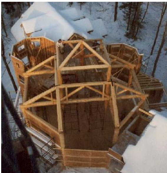
Three-branch and Four-branch Compound Joints
