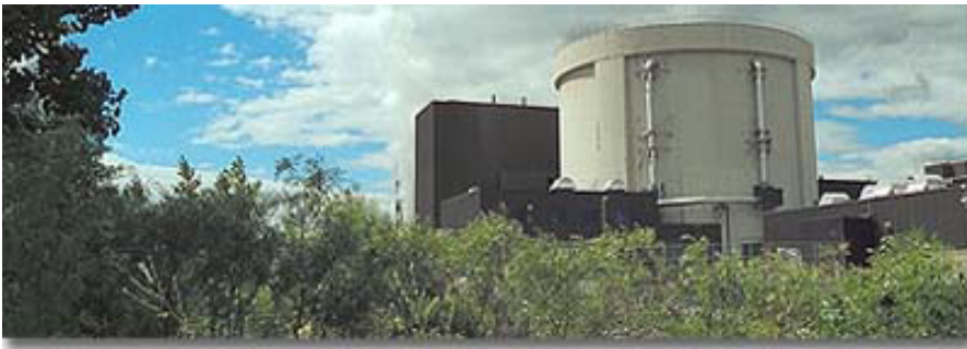
Figure 8. Gentilly 2 Nuclear Generating Station in Becancour, Quebec
