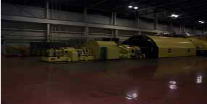
Figure 4. Steel-framed turbine building
