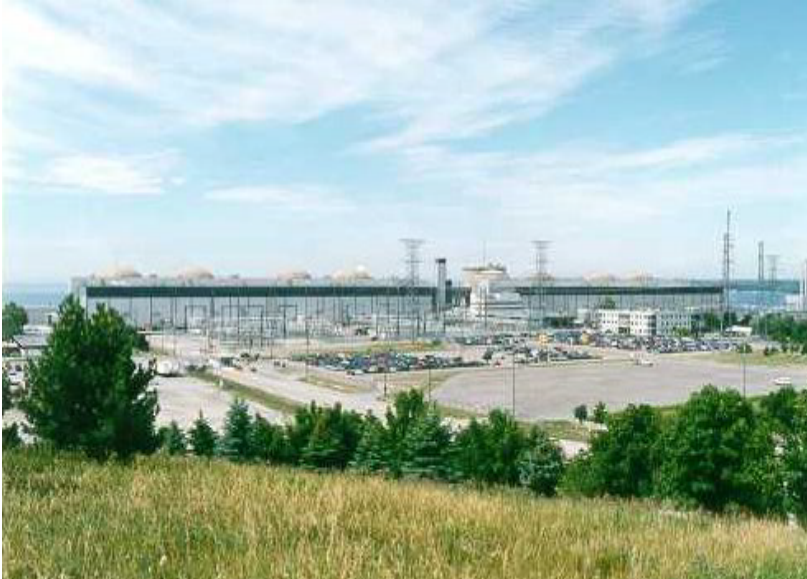
Figure 1. Pickering Nuclear Generating Station in Pickering, Ontario
